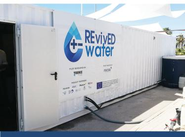
Electrodialysis can also be added as a predesalination step to existing reverse osmosis systems, producing more drinking water from the same amount of seawater with less energy consumption, and at affordable costs. Since May 2019, an industrial-scale pilot plant in Burriana, Spain has been demonstrating this concept.
